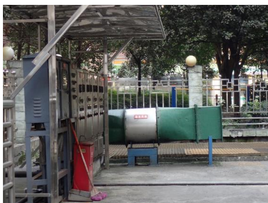
Pump station in Yibin city
