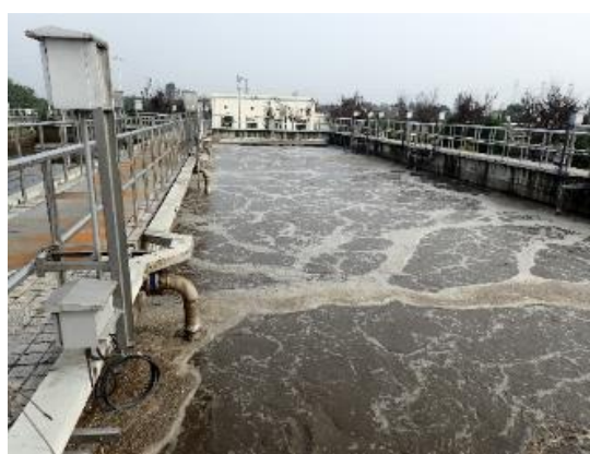
Songya Treatment Plant in Mianyang city
