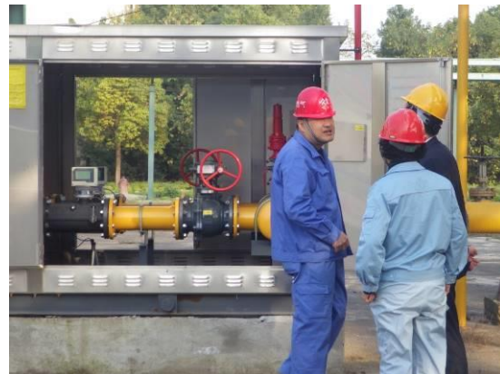
Gas supply regulator station
