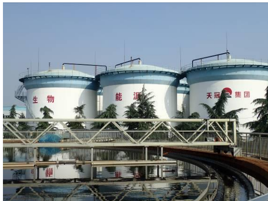
Gas production facilities
