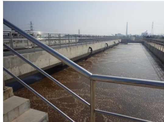
Aeration tank at the South-area Wastewater Treatment Plant (The improved A 2 O process was adopted)
