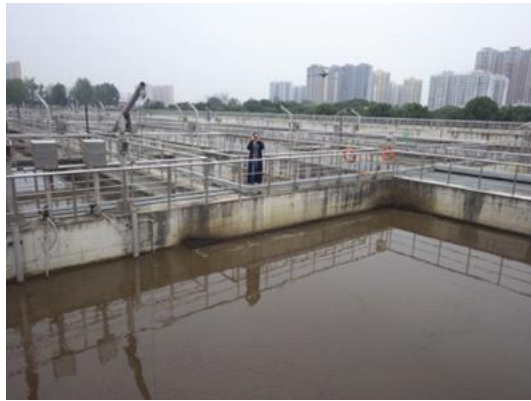
Aeration tank at the North-area Wastewater Treatment Plant (The improved A 2 O process was adopted)
