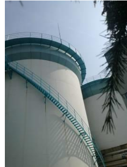
Fermentation tank of the gas production project section at the time of the second survey (March 2018)
