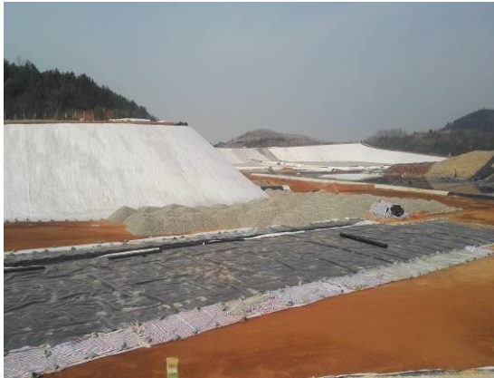
Landfill facility constructed under the Project (Huarong)
