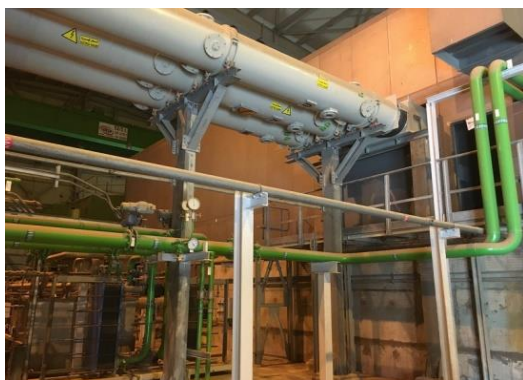
Photo 3: Steam Turbine Room
