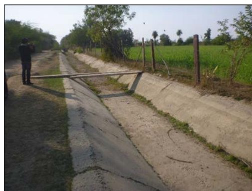
Cleaned canal (section improved by this Project)
