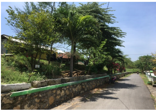
Photo 3: Constructed Levee (Tuban District)
