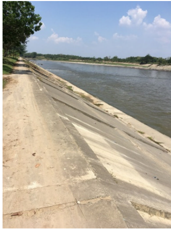
Photo 1: Dyke around Babat Barrage
