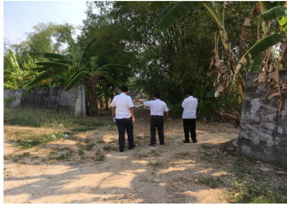
Photo 8: Levee Developed Using BBWS' Own Budget and Undeveloped Area Due to Absence of Land Acquisition
