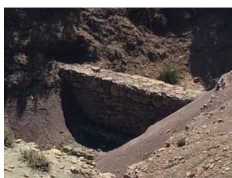
Check dams constructed by the Project (AEF Dam Upper Watershed, Sefrou Province)
