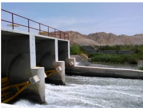
Headwork (Lima Region)
