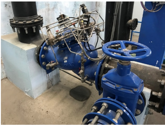
(Left) Valves at a distribution tank connected to SCADA
