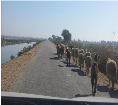
Good condition road Cicar Poole (SH-52)
