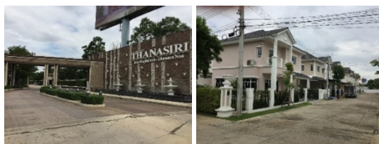
New Housing Project (Thanasiri)
