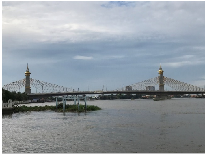
Maha Chesadabodindranusorn Bridge constructed by this project
