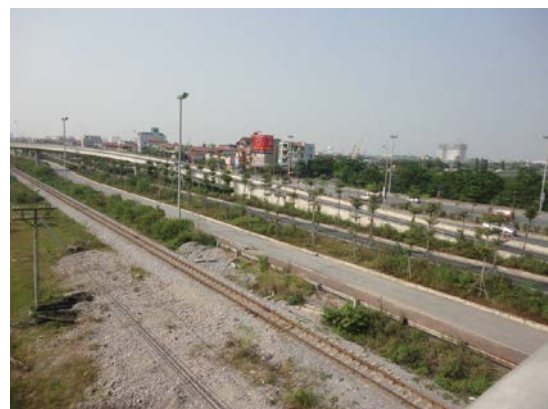
A Part of Clover Leaf Interchange and Rail Road after Realignment
