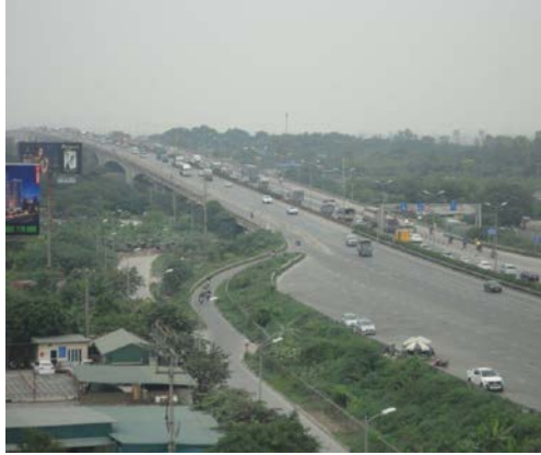
Red River Bridge
