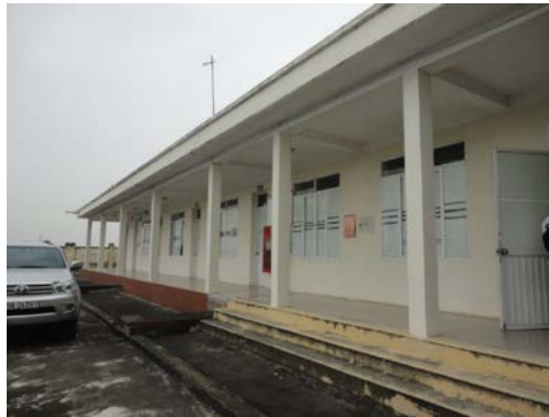
Building of a substation constructed in this project (Yen My Substation, Hung Yen province)
