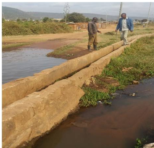
A water canal constructed by members of Kanunka B scheme
