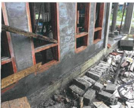
Completed foundation of non-engineered seismic resilient house in Nias District
