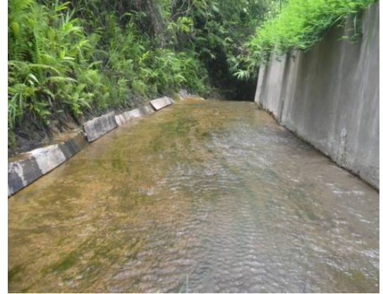
Construction of a headwork under TCP (after the project)
