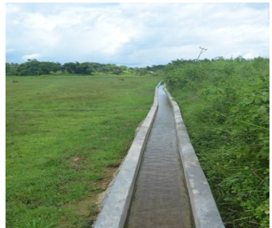
Rehabilitation of a canal under TCP (after the project)
