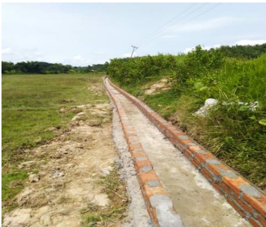
Rehabilitation of a canal under TCP (before the project)
