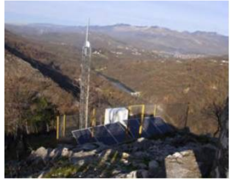
Comprehensive Monitoring System on the Grohovo Landslide
