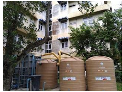
MRB technology in Srinakharinwirot University for greywater treatment and reuse
