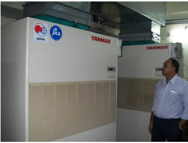
GHP installed in SME in Rajkot
