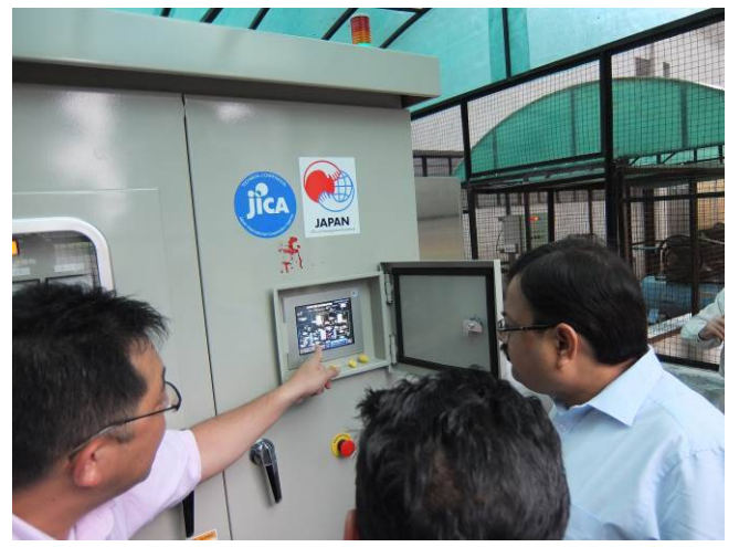
EHP installed in SME in Amul
