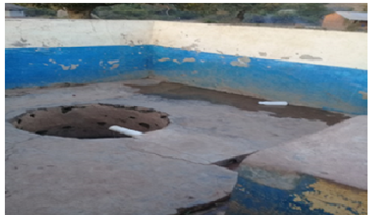
At the Molosiyo Water Point, water tariff is collected, training was done and sanitation is properly managed.
