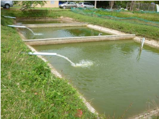
Fish Ponds at Toek Vile Fish Seed Production Station with supplying water by the pump procured under the project
