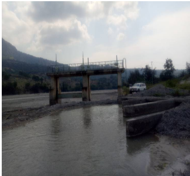
Current Situation at the Intake of Laclo Irrigation Scheme
