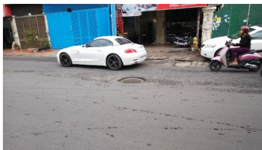
Tuol Svay Prey Area Drainage Area (Manhole sunken by about 5 cm)
