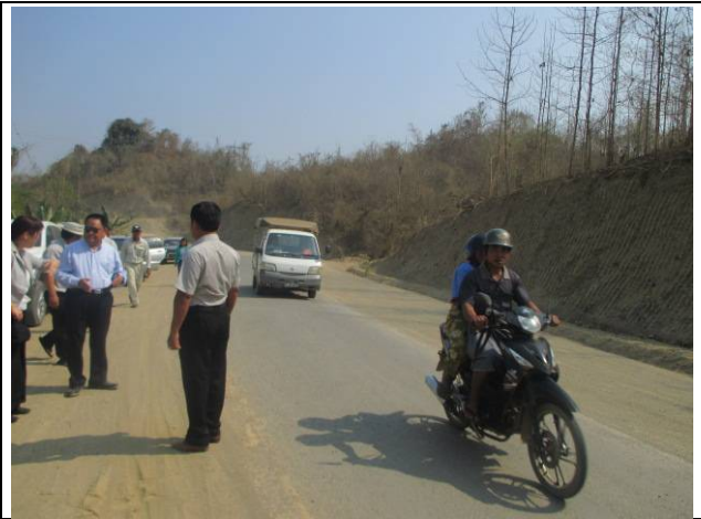
Improved road condition contributes to the better transportation for local people
