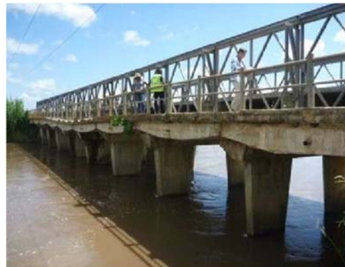
Bridge to be replaced (Document provided by JICA)
