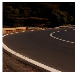
Place where accidents occur frequently (Around Ziba Bridge)
