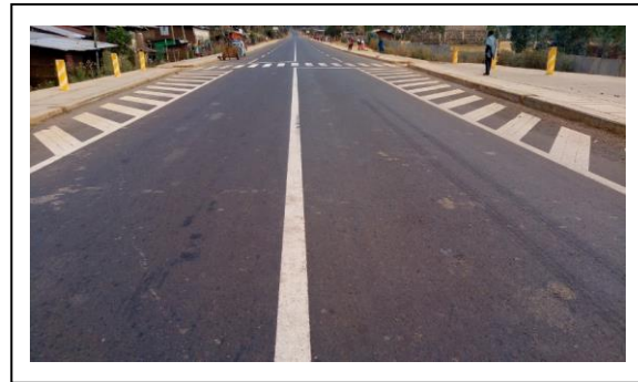
Road rehabilitated by this project (Lumame)
