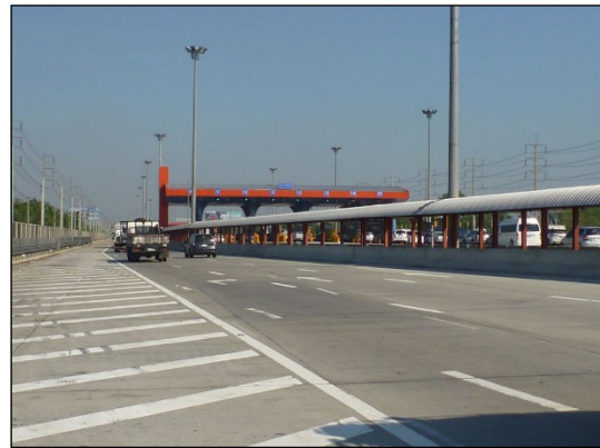
Photo 1: Section surrounding the Toll Station (Out of the Project Scope)
