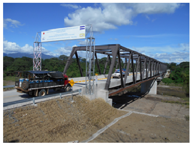
Paso Real Bridge constructed as a part of grant aid of Japan
