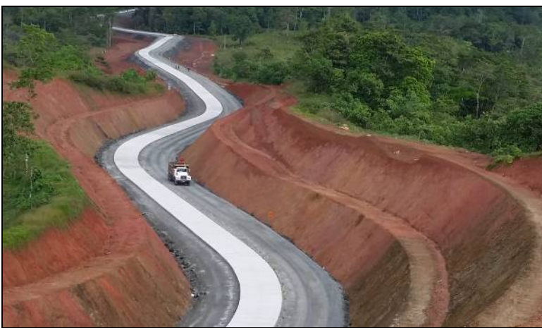
Construction of Nueva Guinea-Bluefields road (135.7 kms)
