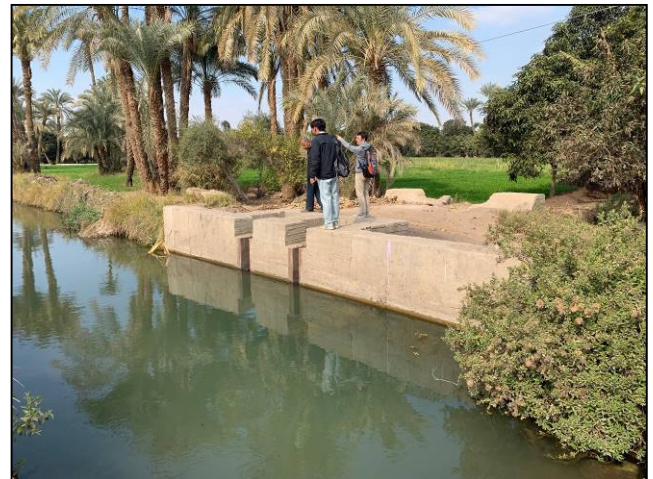
Joint repair works performed by Ebheet BCWUA, in Fayoum, in cooperation with MWRI
