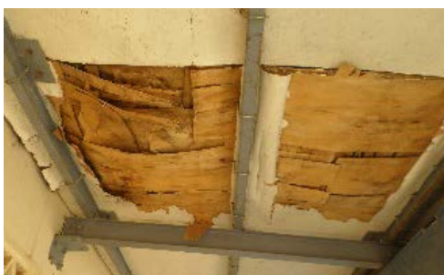
Photo 1: Deterioration of the ceiling due to rain leak
