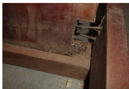
Photo 2: Deflection and cracks of furniture
