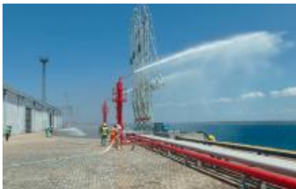
Regular water discharge for inspection of firefighting system
