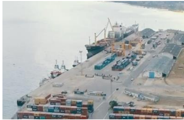
North Wharf (target area of the Project)
