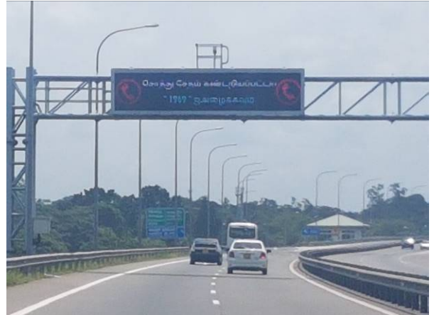
VMS on the Expressway
