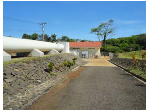
O'Chum No.1 Power Plant (Power Plant Building and Penstock)
