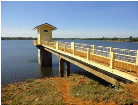
Water Intake Tower of O'Chum No.1 Dam
