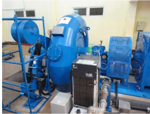
O'Chum No.2 Power Plant (Turbine and Generator)
