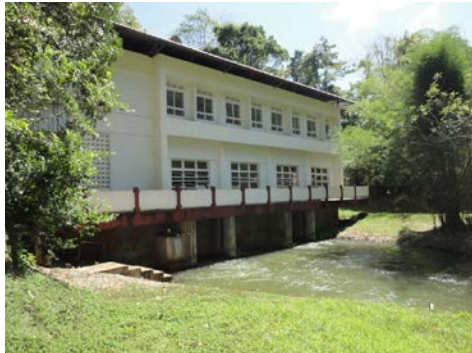
O'Chum No.2 Power Plant (Building)
