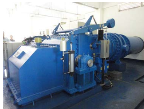
O'Chum No.1 Power Plant (Turbine and Generator)
