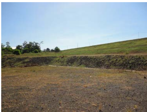
O'Chum No.1 Power Plant (Water Seepage Countermeasure Work)
