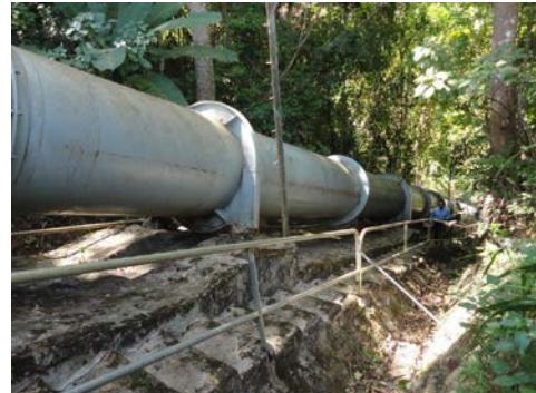
O'Chum No.2 Power Plant (Penstock)
