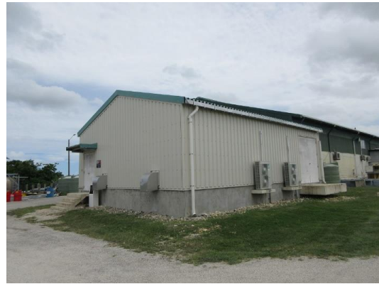
New electrical room at Popua Power Station
