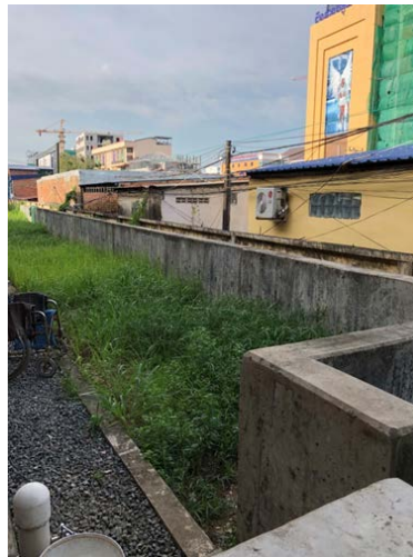
Retaining wall shape at the time of ex-post evaluation
