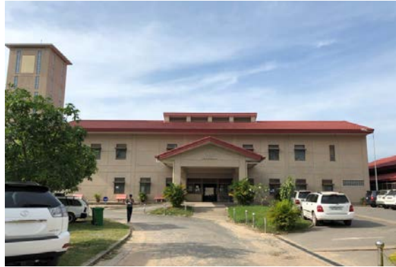
Sihanouk Provincial Hospital (Administrative Building)
