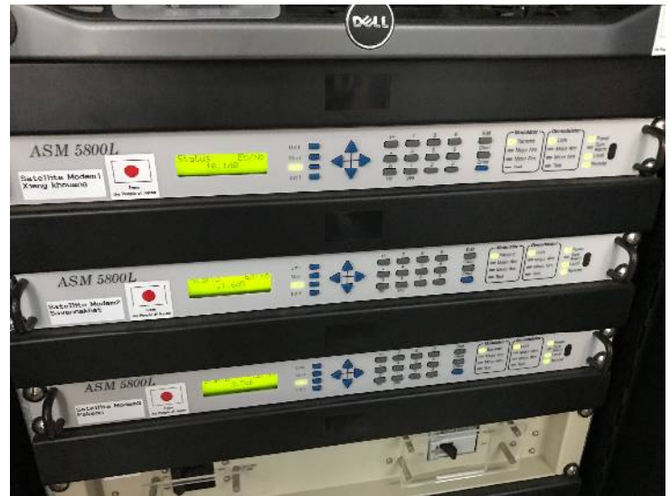
Satellite Modem of each airport
