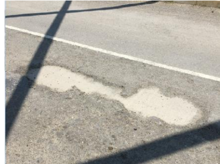
Uneven road surface on Mola Bridge
