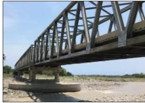
Mola Bridge and reinforced pier and abutment
