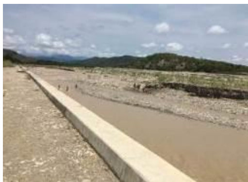
Revetment constructed in the Mola River
