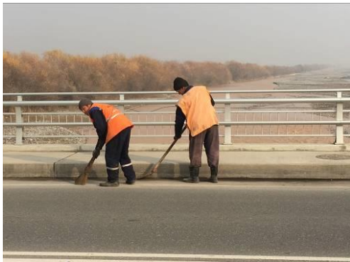
DEU-22 staff cleaning the bridge
