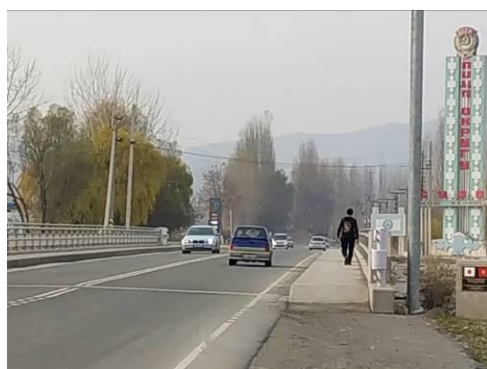
A bridge user on the newly enlarged sidewalk
