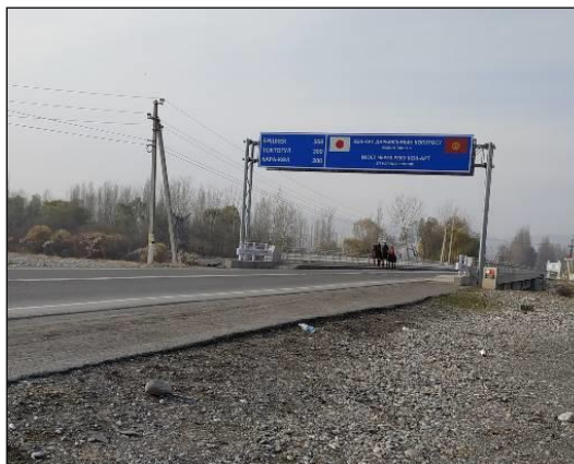
Kok-Art River Bridge and the access road
