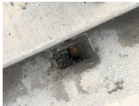
Drainage ditch prior to periodic cleaning
