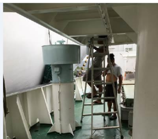
(photo) Maintenance (painting) work
