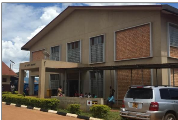
Outpatients Department Building of the Hoima RRH
