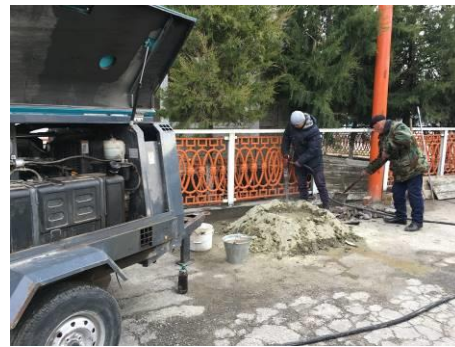
Repairing a road shoulder using an air compressor
