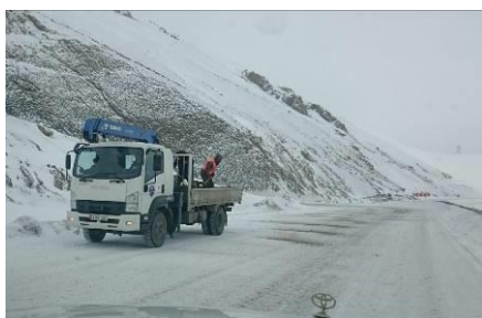
A worker spraying snow-melting salt and sand
