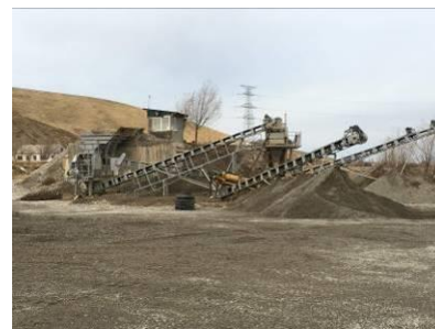
An aggregate plant
