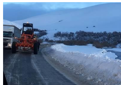
A rotary blower removing snow on a mountainous road
