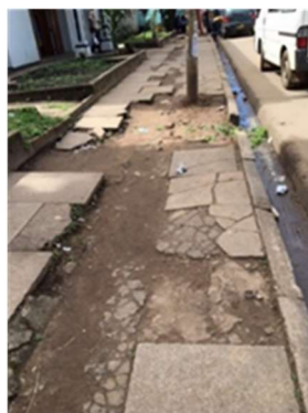
Footpath in Livingstone Av. (section 5)
