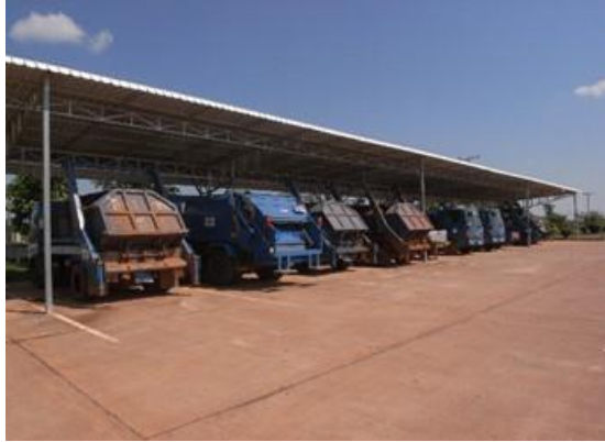
Photo 2. Solid waste transfer station in Vientiane (compactor trucks and skip loaders on standby after waste collection for the day)
