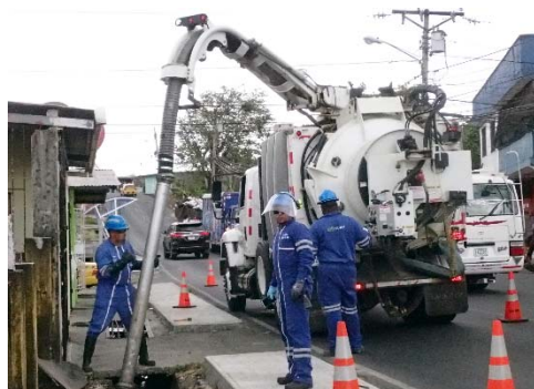
SOAP staff fixing the clog in sewage
