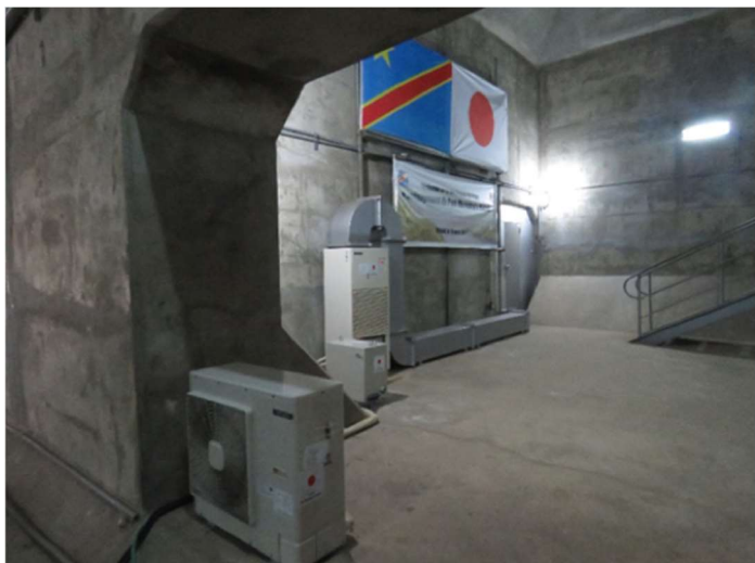
Injection dry air system machine (GA)
