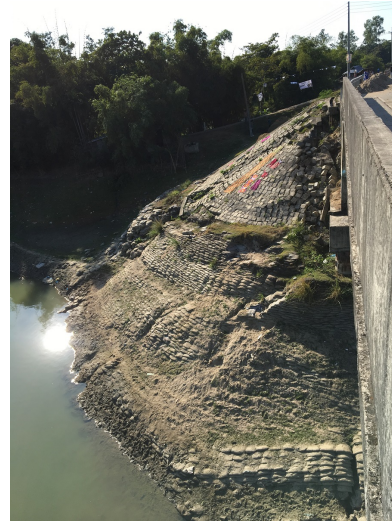
Damages to the slope protection (R280-038c Bridge)
