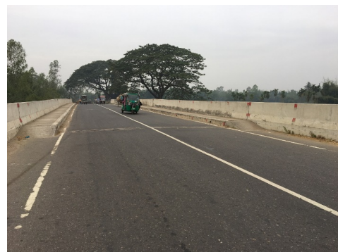
A bridge developed through this project Bridge 106a on National Highway No.4 (Dhaka Zone)
