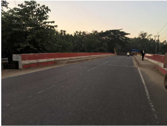
N1-394e Bridge (Chittagong zone)
