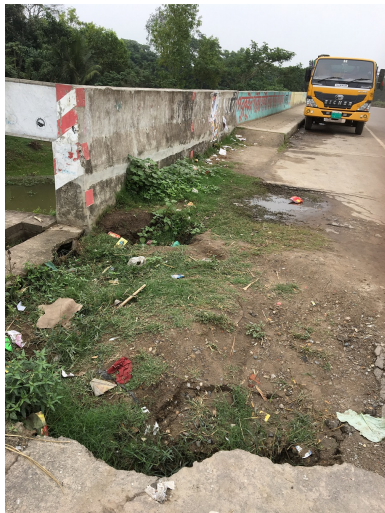
Damage between the approach road and the abutment (N102-035a Bridge)
