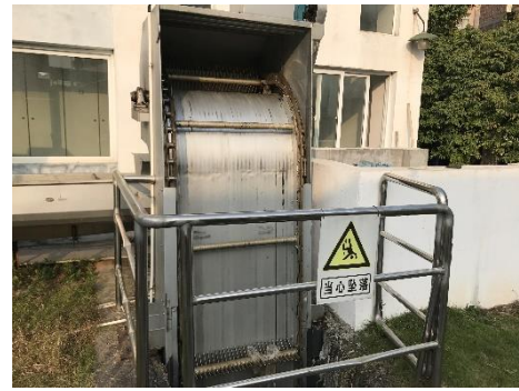
Nanmentang Embankment Sewage Pump Station (coarse screen)
