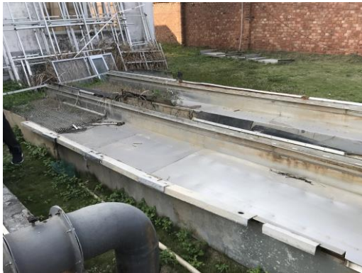
Damaged coarse screen
