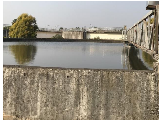
Deteriorated part of concrete structures
