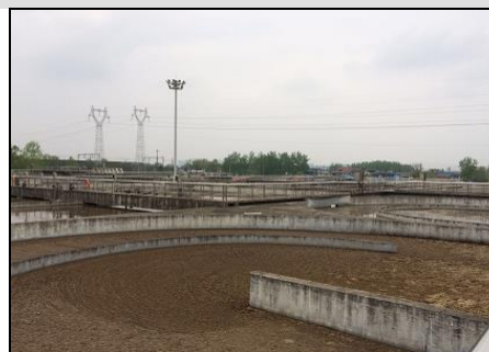
Reaction tank at the Bengbu Sewage Treatment Plant No. 2, which was developed in this project
