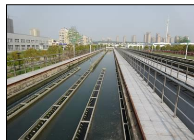
Sedimentation basin of the 1 st purification plant of Bengbu Zhongyang Environment & Waterworks Co., Ltd., Huaiyuan County, constructed in this project
