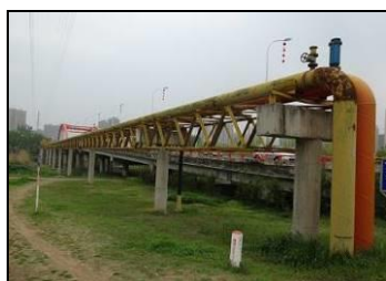
Sewer pipe in Wuhe County, which was installed in this project
