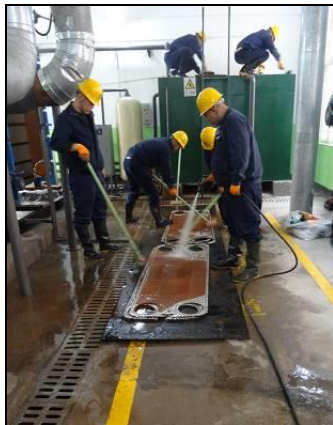
Periodic maintenance of the heat transfer plates at a heat exchange station developed by the project
