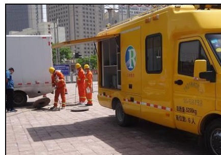
Maintenance of the heat supply pipes developed by the project
