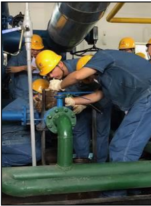
Technical training at a heat exchange station developed by the project
