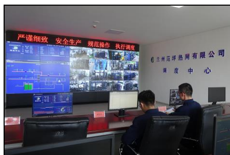
Lanzhou Fanping Thermal Network Co., Ltd.'s control station developed by the project
