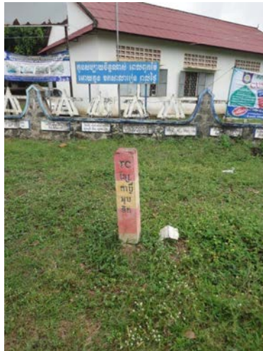
Marking post (The optical cable is buried under this)
